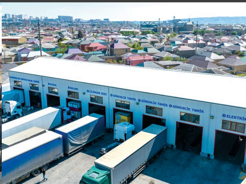
Binagadi truck park Sandwich panel
