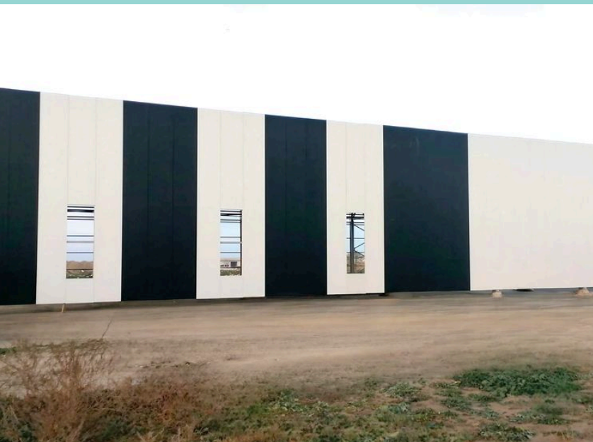
Bafco footwear factory, Aghdam Sandwich panel
