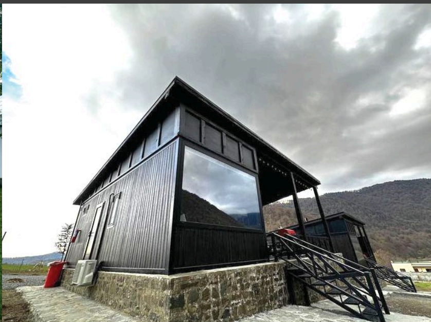
Runaway House Container
